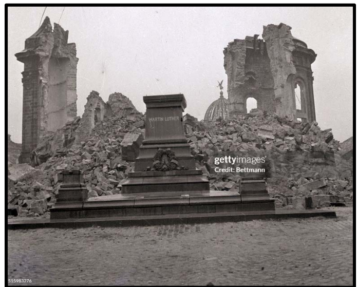
This is the first of two photos of the ruins of the Frauenkirche (see photo, page 9, and map, page 2). At the front is the base or pedestal for an 1885 statue of Martin Luther, which was later restored and returned to the site. The date of this photo is given as March 16, 1946, 13 months after the firebombing of the city. Two major remnants of the Frauenkirche structure stand among the rubble, and the dome of the Dresden Academy of Fine Arts is seen in the background (Getty Images).
